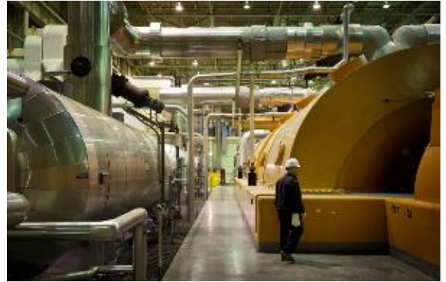
Terry Pickens, director of nuclear regulatory policy for Xcel Energy walked by one of two steam powered generators at the plant. Steam is heated in the nuclear vessel. The Xcel Energy Prairie Island Nuclear Plant north of Red Wing is looking to boost electrical output at the plant.
